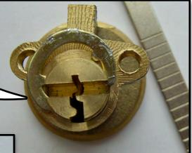
THE CIRCLIP HOLDS THE PLUG IN PLACE. HOWEVER EVEN WITH THE CIRCLIP REMOVED THE PLUG WILL NOT COME OUT **BECAUSE** THE PINS ARE STILL BLOCKING THE **REMOVAL** OF THE PLUG
